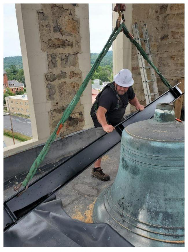
Times Observer Photo by Brian Ferry The 11 original bells — cast in 1926 — were removed from the wooden frame that formerly held them in place and a new steel frame was hauled up by the crane.
